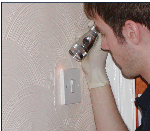
• Remove and inspect light switch covers
